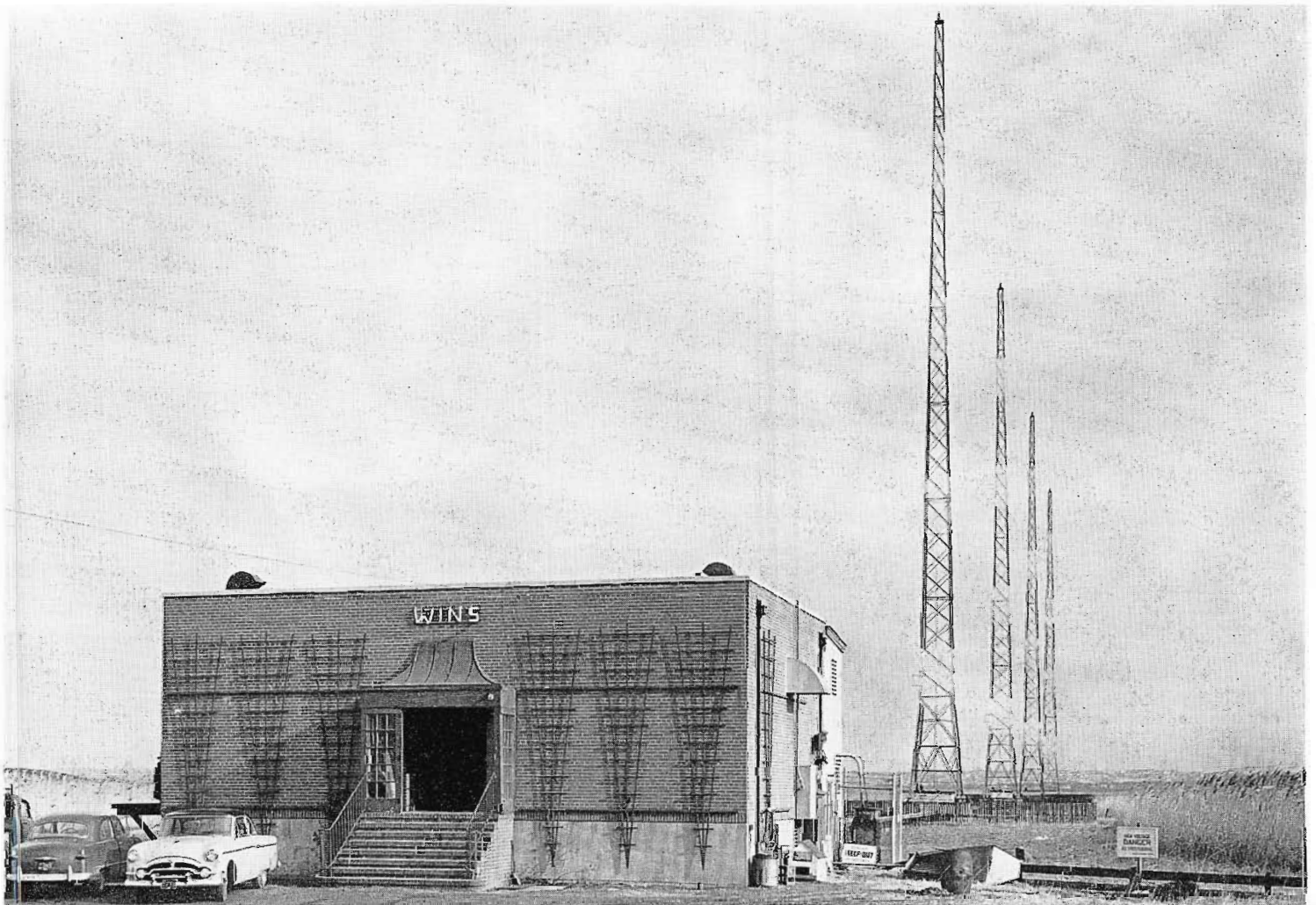
FIG. 7. This is the WINS transmitter building in Lyndhurst, New Jersey. The antenna system is directly behind the building.
