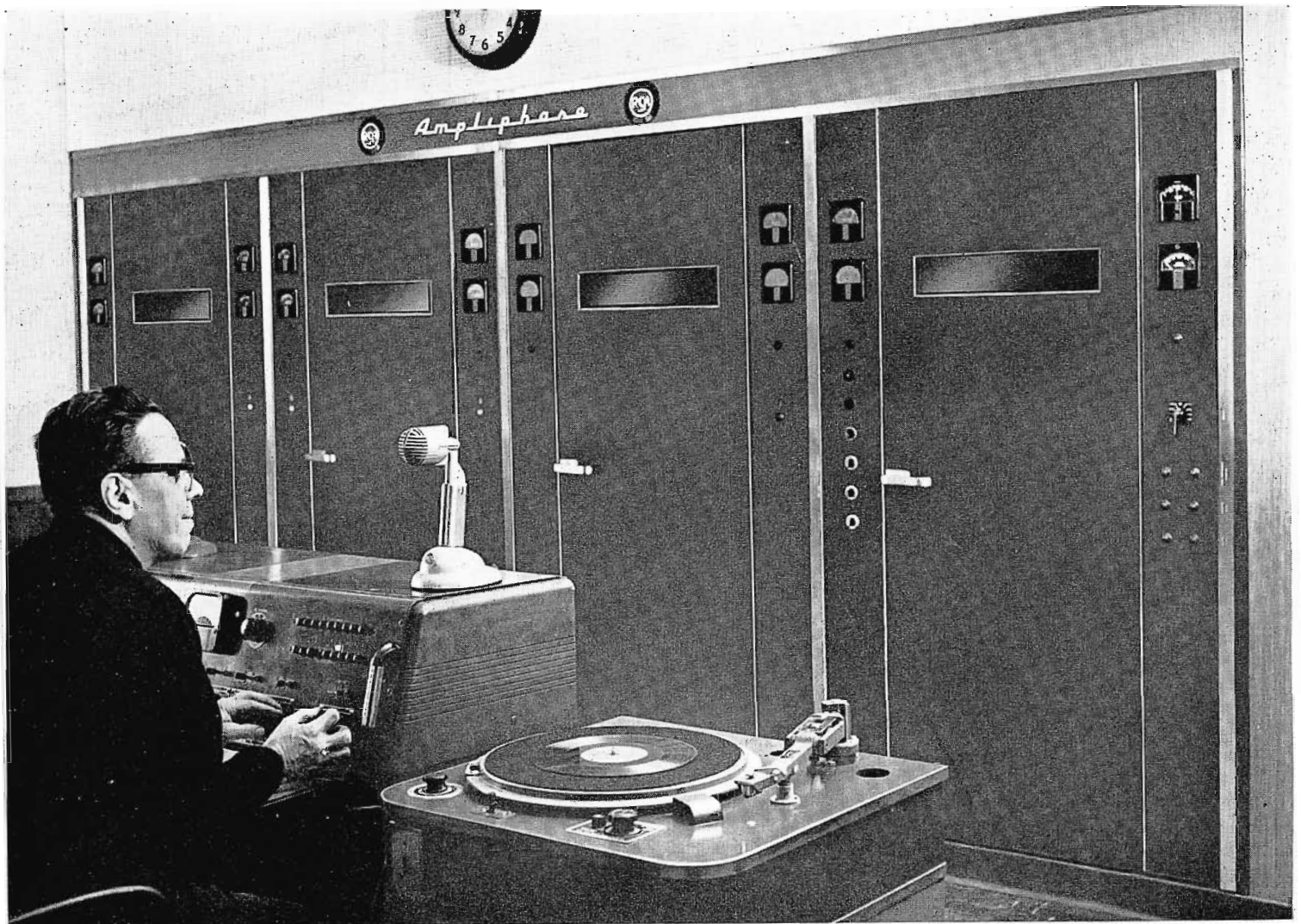
FIG. 10. Alfred Jorgenson, WINS Transmitter Engineer, is shown at the 76B Console in the transmitter building. One of the 70C Turntables is on his right. The input and monitoring equipment is to the rear within arm's reach. This console and turntable can be used to originate programs at the transmitter site.
