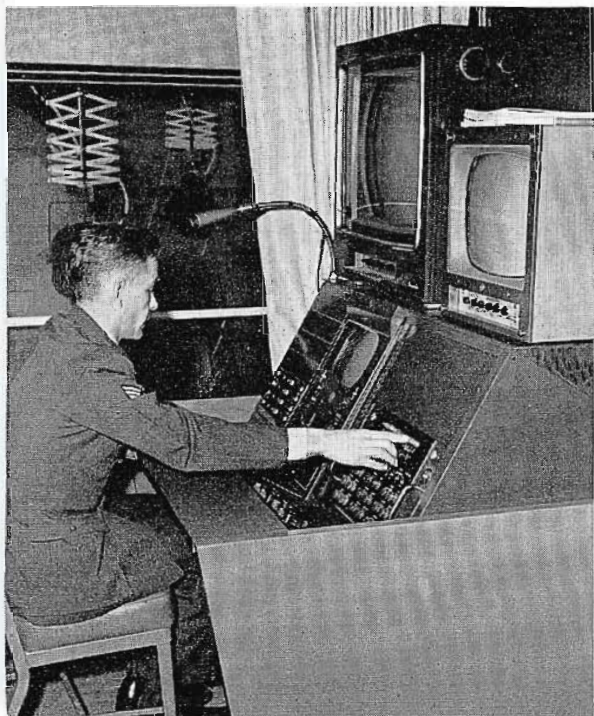
FIG. 7. Film-room operator controls film and slide output from this control console. Atop console are a 17-inch program monitor and a 21-inch on-air color monitor. Film room is in glassed-in balcony area above map room.
