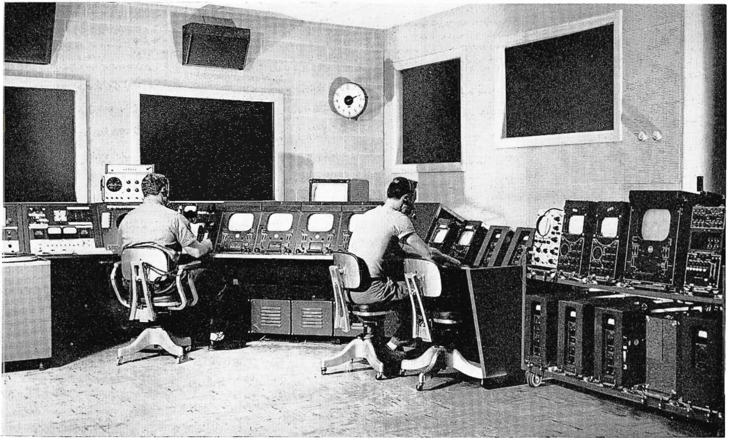
FIG. 13. Master control is located so that operator can see into both studio control rooms, both announce booths, and the projection room.
