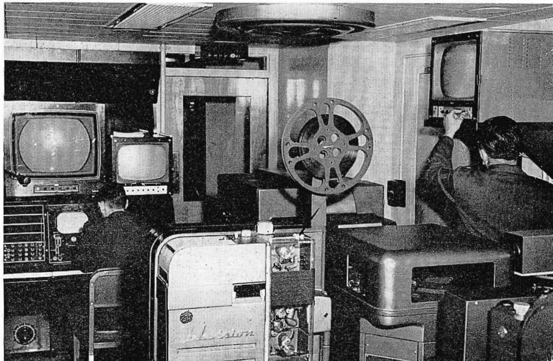
FIG. 8. The film room at SAC includes an RCA color film chain, 16mm film projector, 35mm slide projector and multiplexer. Films and slides, interspersed in briefing program schedule, educate SAC command in various fields of military knowledge.
